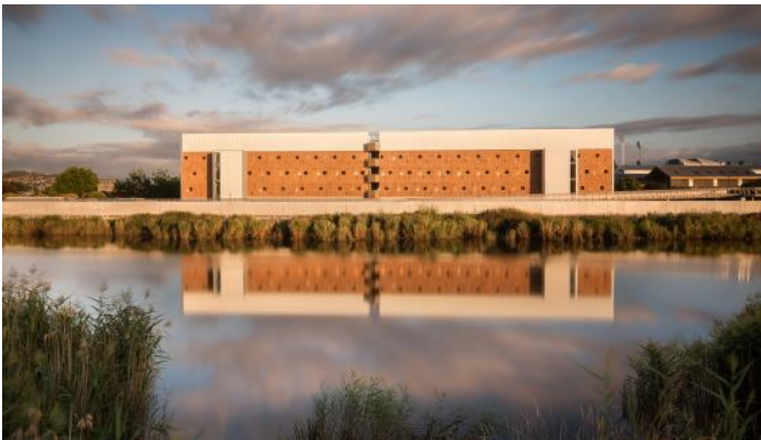
Inveresk Student Accommodation, University of Tasmania 2 Invermay Rd, Launceston TAS
