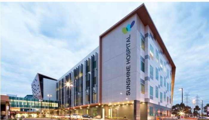
Sunshine Hospital – Acute Services Building Furlong Rd, St Albans VIC
