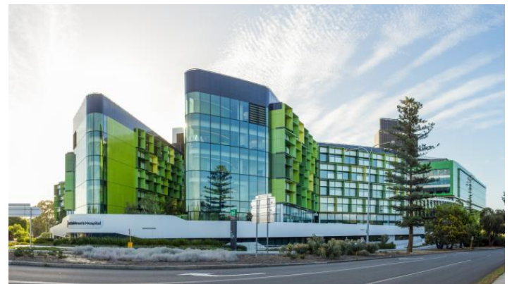
Perth Children's Hospital 15 Hospital Ave, Nedlands WA
