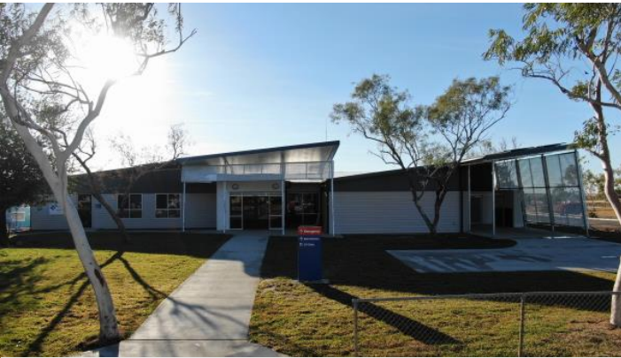
McKinlay Shire Multi Purpose Health Service 1 Burke St, Julia Creek QLD
